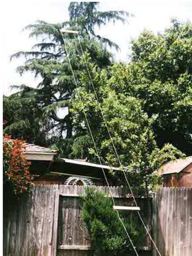
Configuring the FFD requires only the positioning of the two legs. The feeder portions of each of the two legs run from the antenna tuner to a center insulator, with the wires roughly parallel to each other and about six inches apart. On the lower HF bands, even wider spacing between the feeder portions of each wire won't degrade performance. From the center insulator, the remainder of each leg runs outward in opposite directions, producing the flattop portion.
